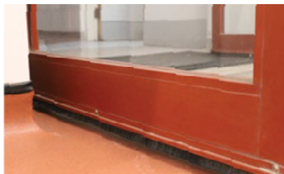
Figure 10. Example of a door adequately pest proofed with brush strip
