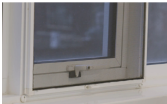
Figure 11. Example of a window adequately pest proofed with an insect screen
