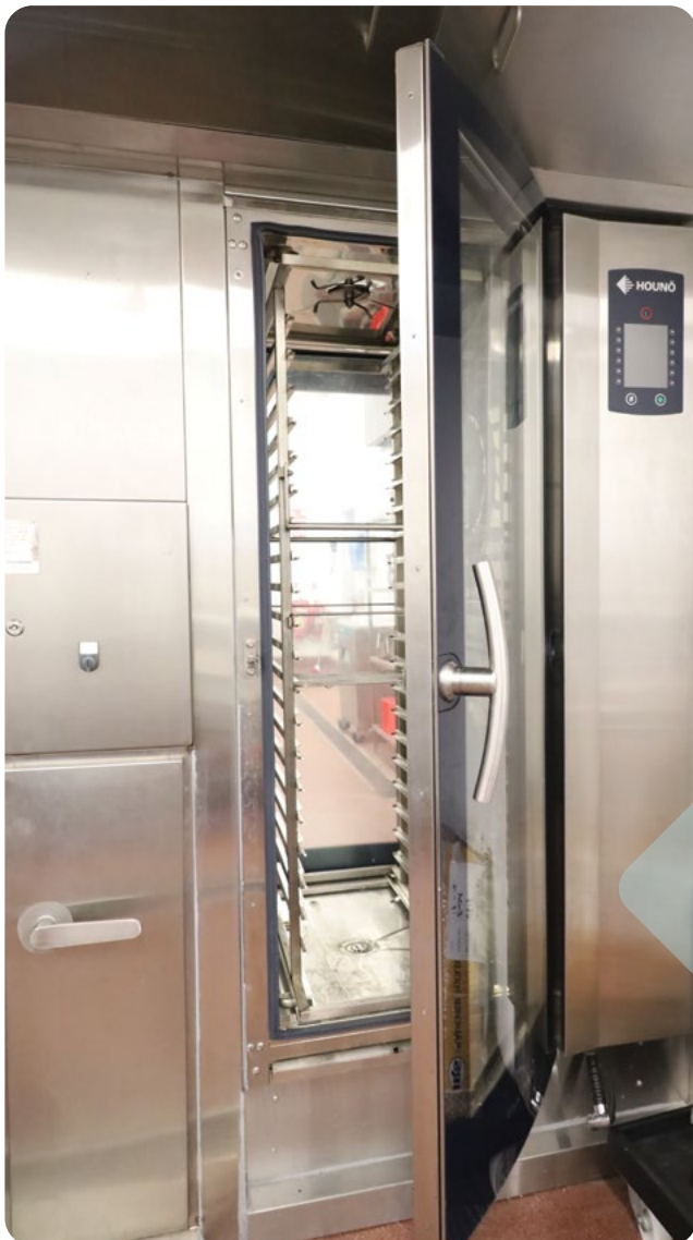
View from raw meat area, through double-door cooker to cooked meat area.
